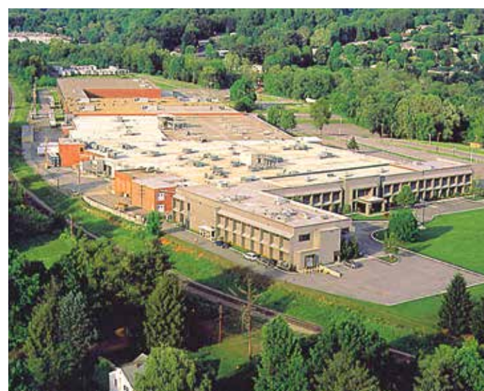
AERUS MANUFACTURING PLANT | BRISTOL, VA
